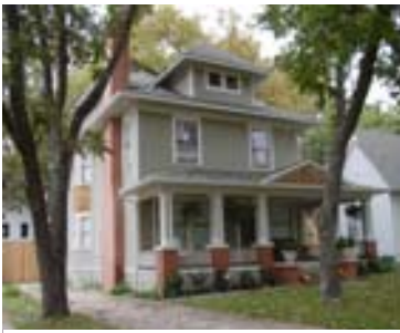
Prairie house in the Vickery Place Neighborhood
