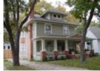
Prairie house in the Vickery Place Neighborhood
