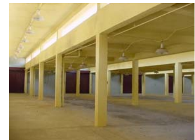
Sheep & Goat Barn Interior After Restoration
