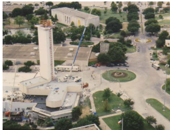
Lifting Re-created Eagle to Top of Tower
