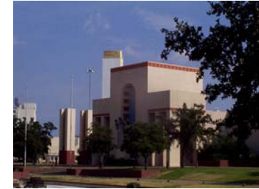
Automobile Building Portico – After Restoration
