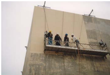
During Restoration (Applying Keim)
