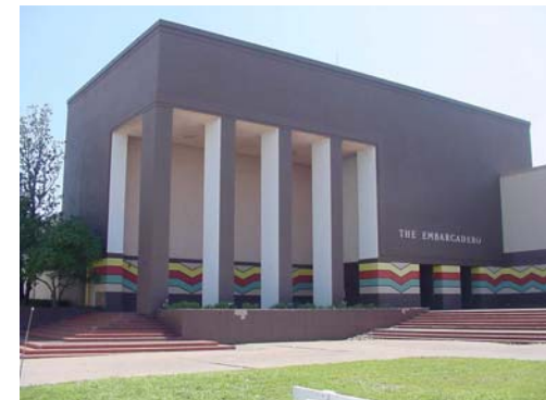
Embarcadero Building- Existing
