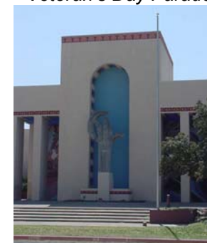
Automobile Building Portico - After Restoration
