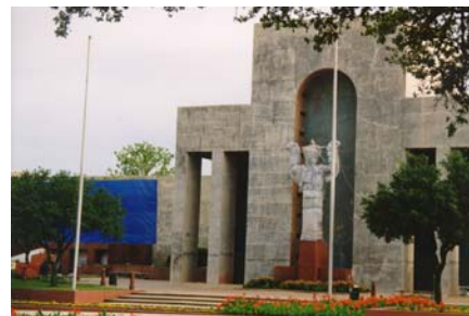
During Restoration (After cleaning)
