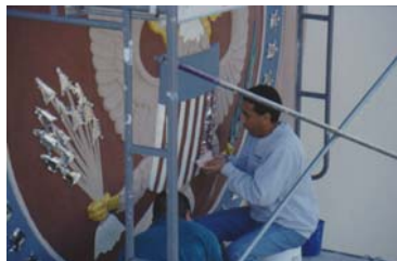
Restoration Work on Medallion
