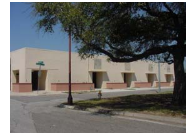
Sheep & Goat Barn After Building Restoration Before Mural Re-creation
