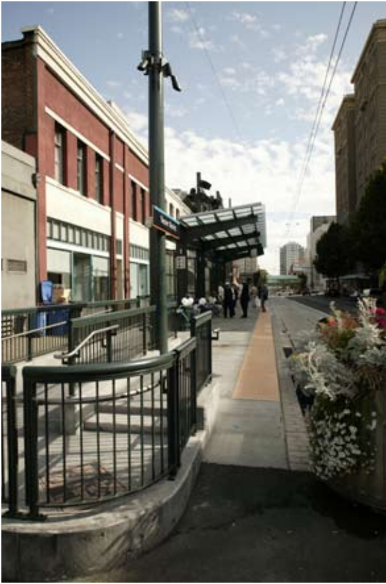
The city of Tacoma streetcar station provides a pedestrian shelter with disability access.
