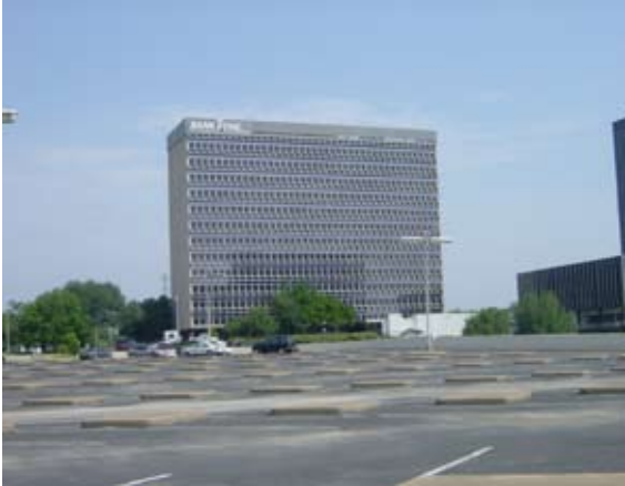
Large surface parking lots produce an overwhelming amount of storm water because of their limited absorption capacity. The run-off from roads and parking lots picks up oil and pollutants which concentrate in the municipal water collection system.
