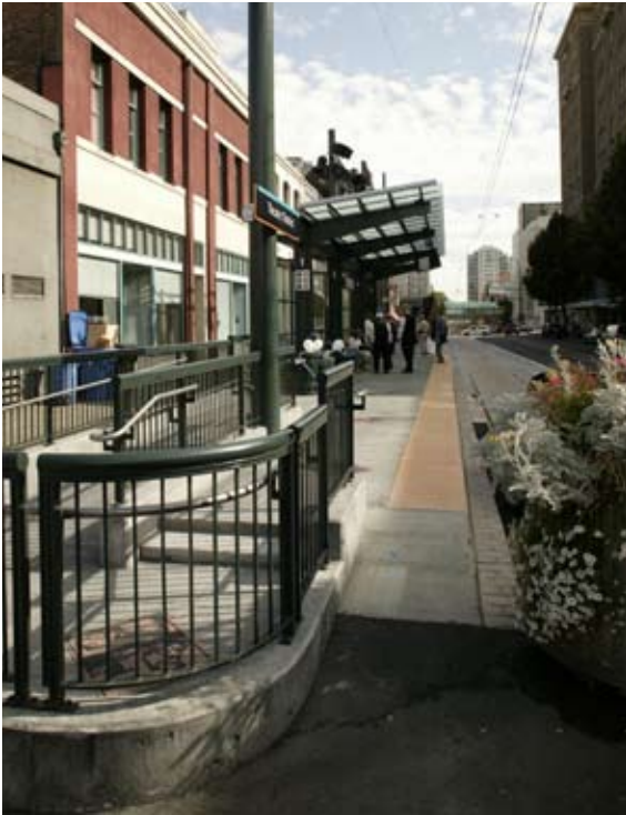
Mixed-use zoning in station corridors will attract activity day and night, helping maintain safety and vibrancy.
