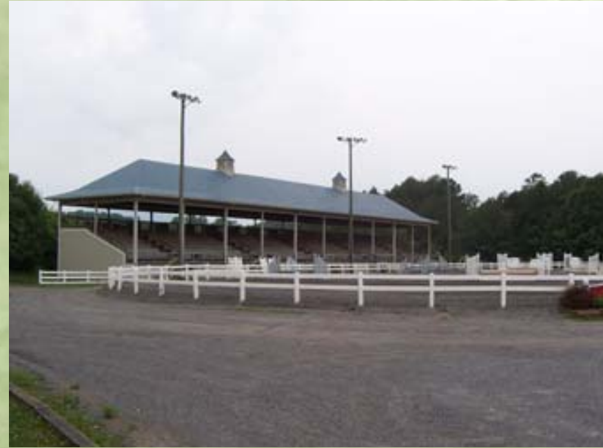
Virginia Horse Center Covered Grandstand Seating
