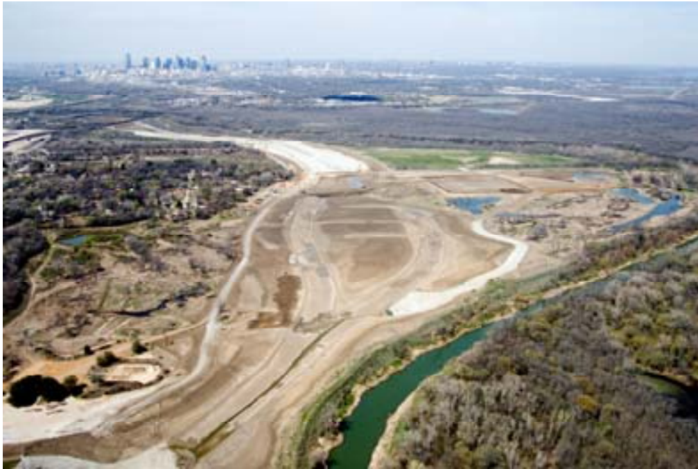
Cells E, F and G, looking north from Loop 12, into what used to be the Sleepy Hollow Golf Course
