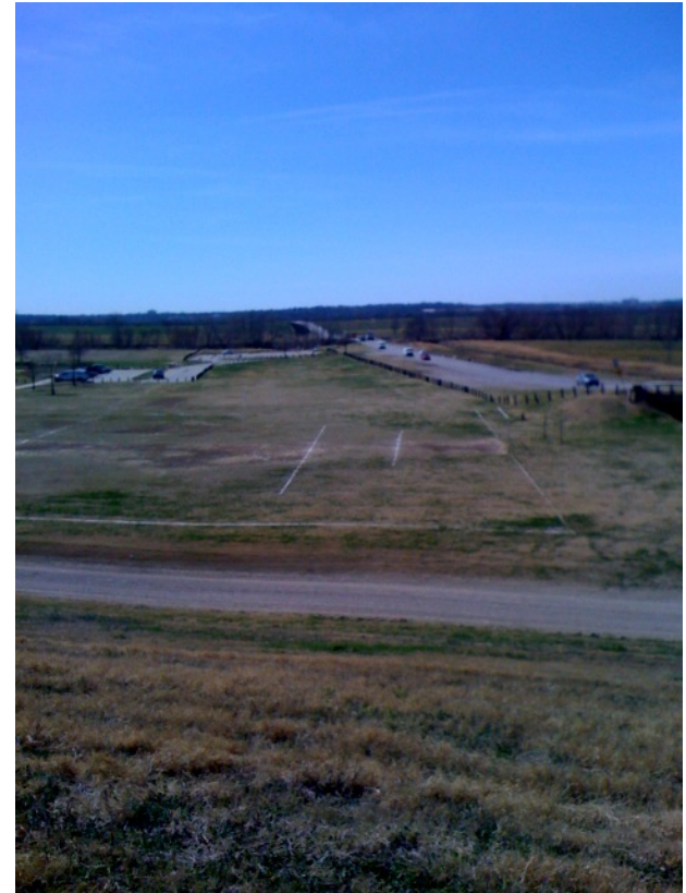
Sylvan Bridge looking south
