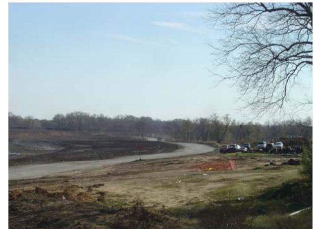
Lower Chain of Wetlands Construction Site
